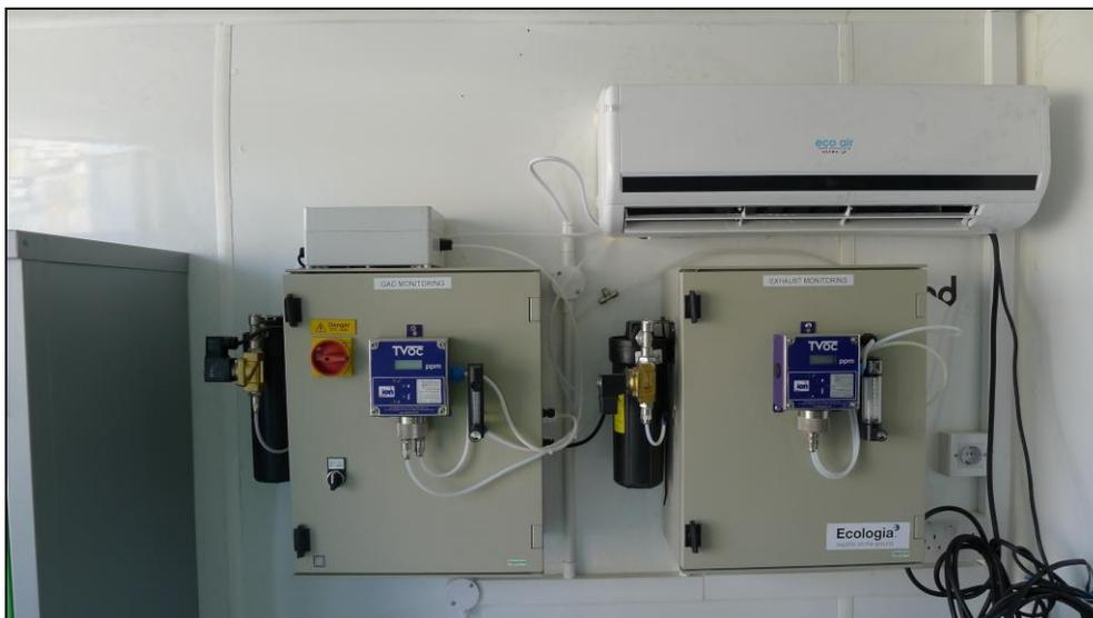
*Ecologia's in-house designed and built automated VOC monitoring and datalogging system*
