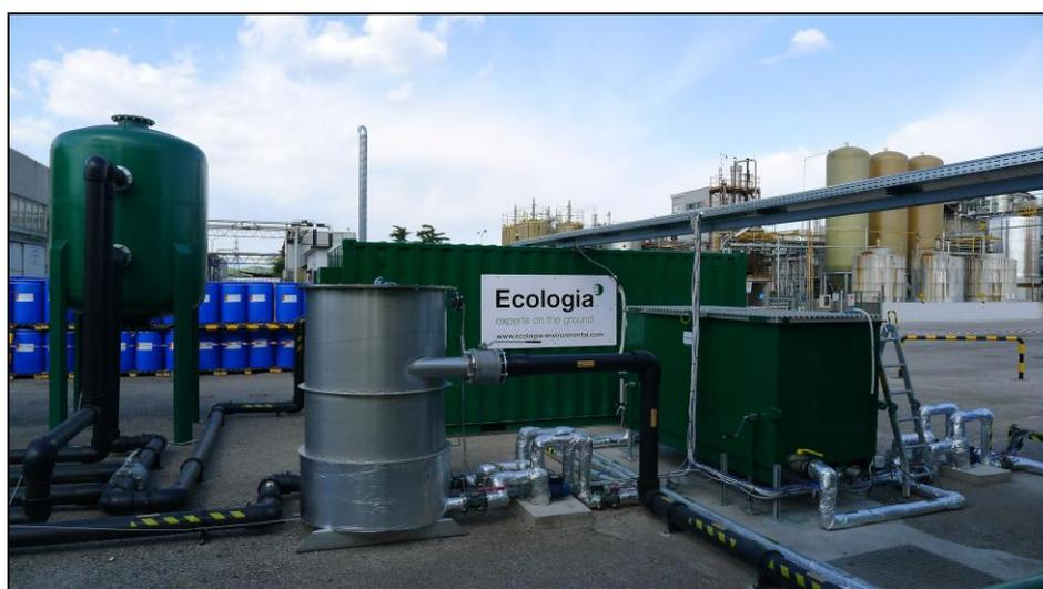
The MPE system applies a system flow rate of 1000 m<sup>3</sup> air per hour at a vacuum of approximately 500mb (gauge pressure) to the subsurface, removing liquid and vapour via 2" drop tubes ('slurper pipes') positioned into 3" wells drilled to either 8m bgl or 12m bgl to intercept the perched water systems. The wells are operated in a cycle to allow repeated alternation of the sub surface thermodynamic system, thereby
