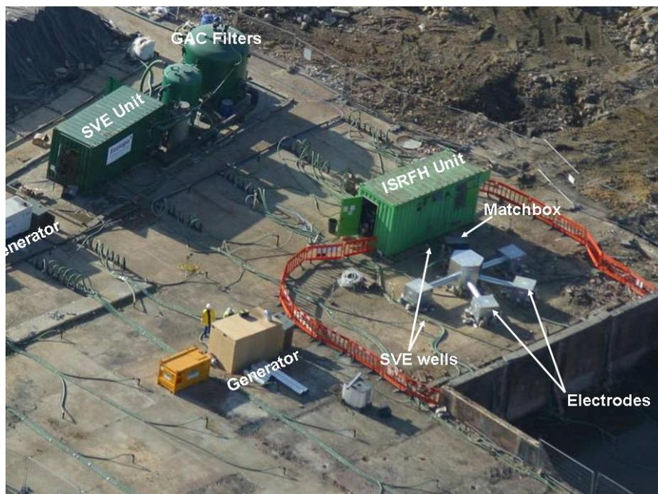
Figure 1. Aerial photo of the ISRFH remediation layout during a remediation project.
