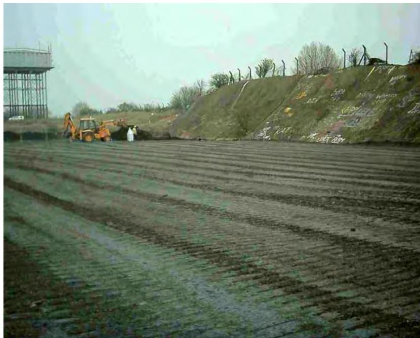
Plate 7.1: Biopile base following completion
