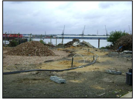
Groundwater ozone sparging container and sparging wells on site.
