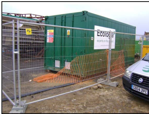
Groundwater ozone sparging container and sparging wells on site.
