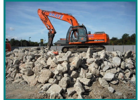
Breaking up the concrete hard standing across site.
