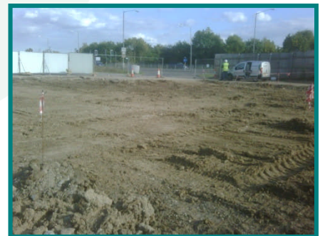
Former Chestfield Service Station upon completion of remedial works
