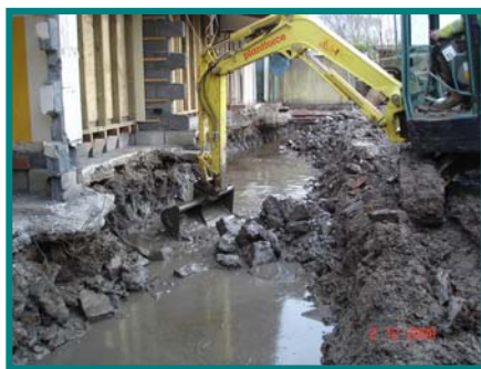
Sorting / segregation of material within the excavation. Rear of bungalow removed.
