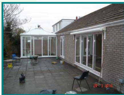
Rear of bungalow re-built on completion
