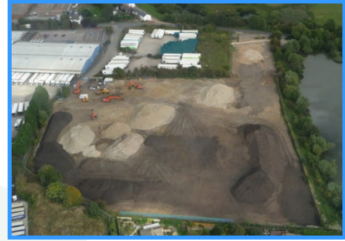
Faversham Foundry Post Remediation work.
