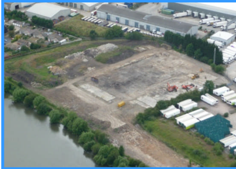
Faversham Foundry Before Undertaking Remediation work.
