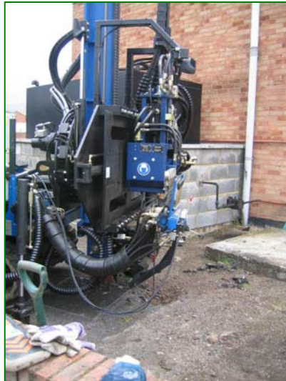
Installation of the Sparging wells
