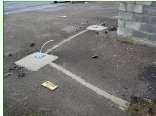
Sparging wells during installation works
