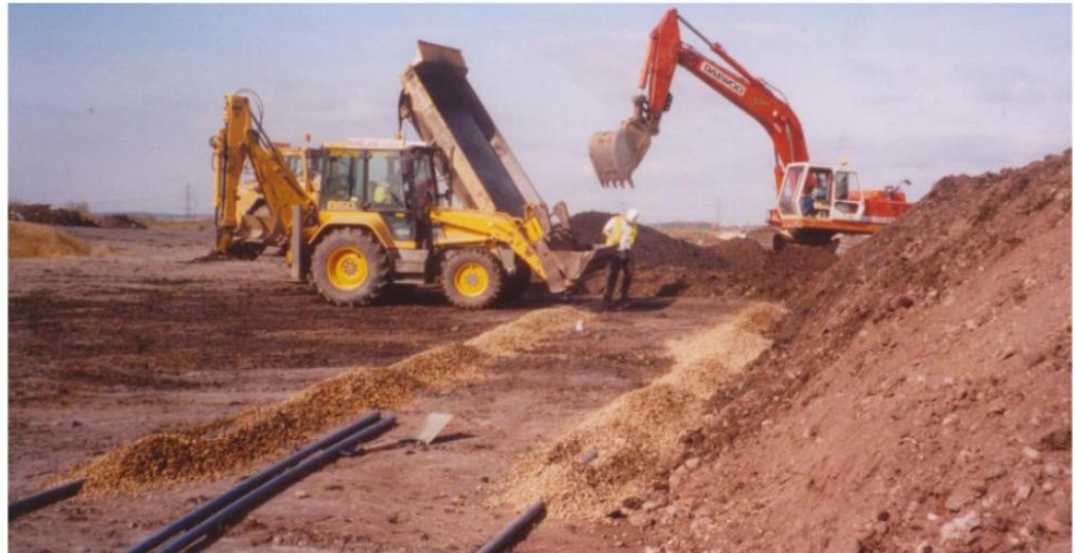
Plate 7.2: Biopile formation works
