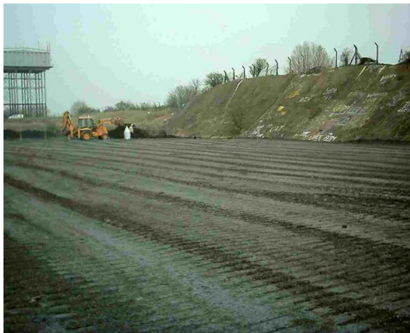
Plate 7.1: Biopile base following completion
