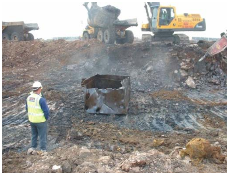
Plate 6.2: Supervision of the excavation process
