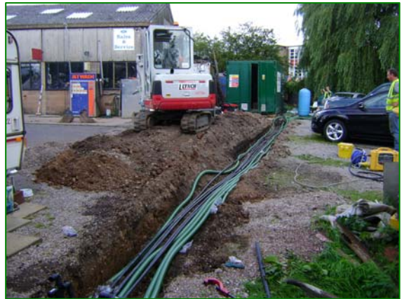
Installation of the gas distribution and SVE lines
