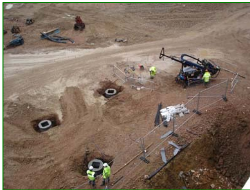
Installation of the extraction wells by Ecologia's drilling division
