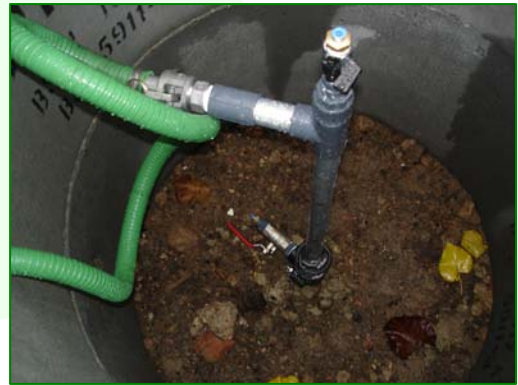
Slurper Well Head
