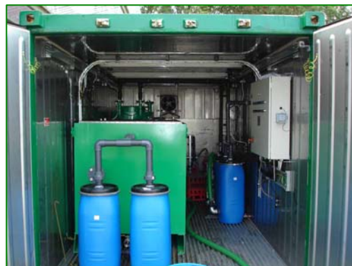
Containerised automated treatment system manufactured by Ecologia in Kent
